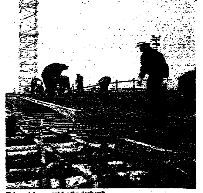
Fixing reinforcement for the deck unit
